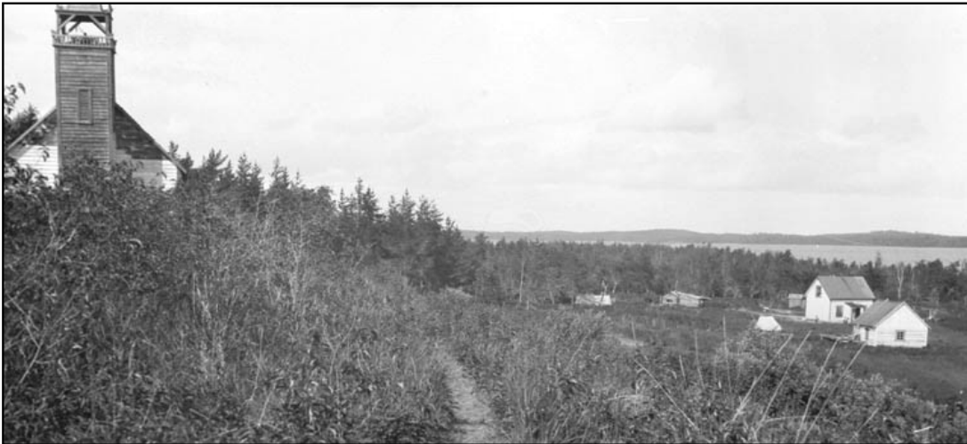
The back of the Osnaburgh House property circa 1929 with the church overlooking the grounds of the trading post. (National Archives of Canada)
