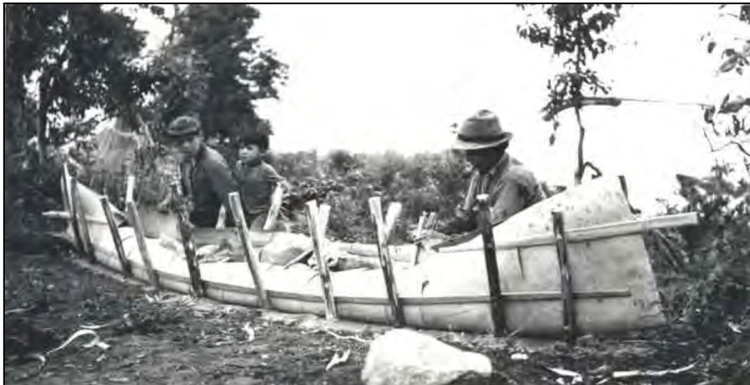
Construction of a birch bark canoe at Osnaburgh, circa 1883. (Photo by R. Bell, National Archives of Canada)
